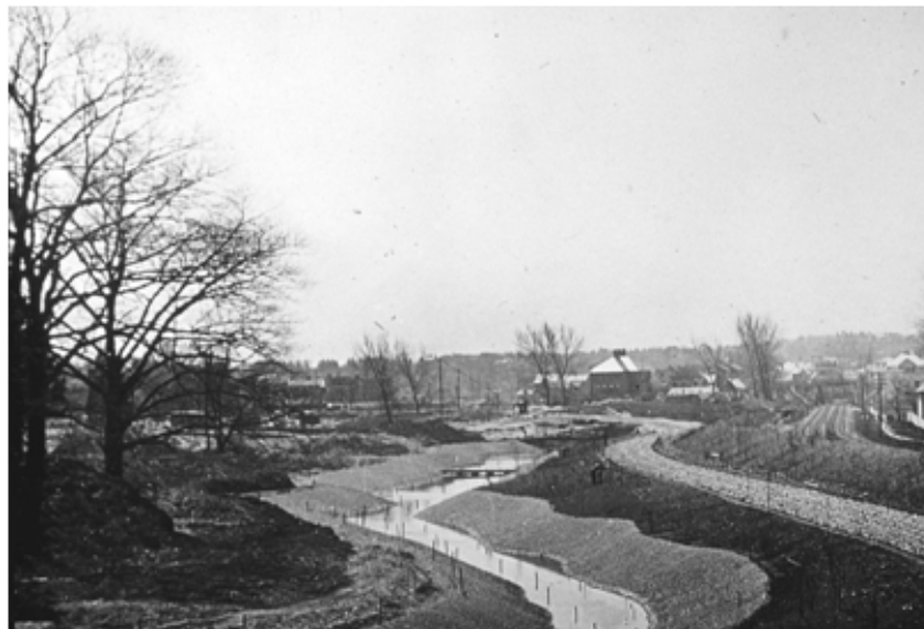
Figure 4.7. The Muddy River Improvement Project, c. 1890, showing the construction and grading of the Riverway. Source: Frances Loeb Library, Graduate School of Design, Harvard University.
