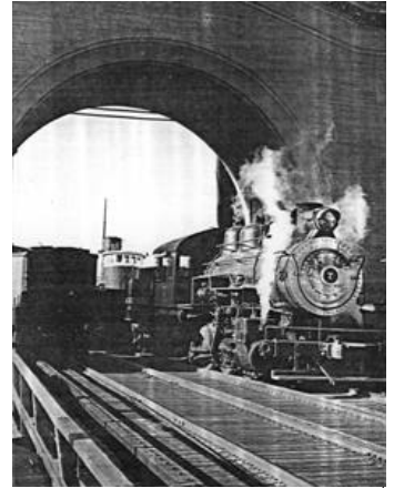
24 The ferry slip that still exists on the site
