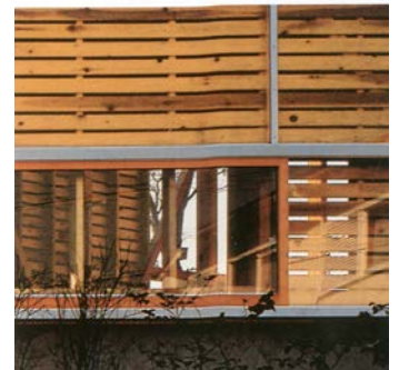
8 House in Kobe, Japan by Go Yoshimoto features prefabricated facade made of metal panels and wood slat panels
