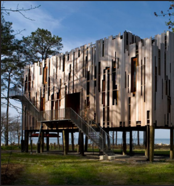
Loblolly House ————— Wood Slats Kieran Timberlake, 2007 Chesapeake Bay, Maryland
