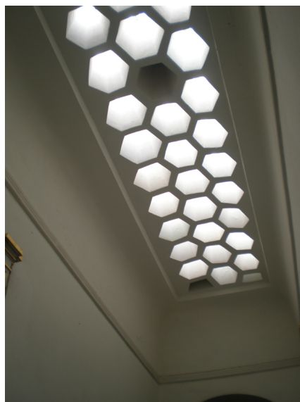
Skylights in Topkapi Palace, Istanbul
