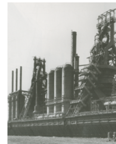
FIGURE 2.2 Andrew Garn Blast Furnace A and B with dismantled powerhouse in foreground, 1993 Photograph unknown dimensions in Bethlehem Steel: Princeton Architectural Press, 1999
