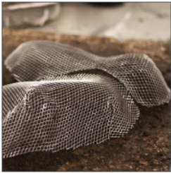
REBAR MESH IS ADDED OVER THE CONTOURS OF EXISTING DIRT MOUNDS
