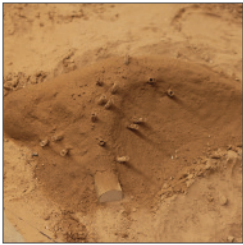
LIGHT TUBES AND DOOR FRAMES ARE ADDED TO AN EXISTING SAND DUNE
