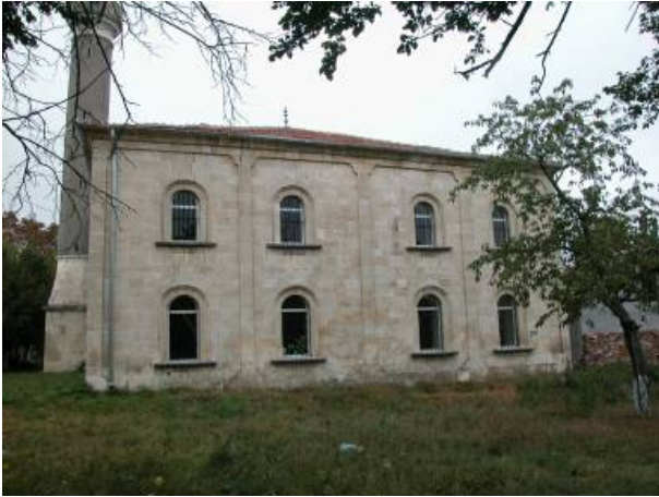
Rear of mosque. Note faux columns and capitals.
