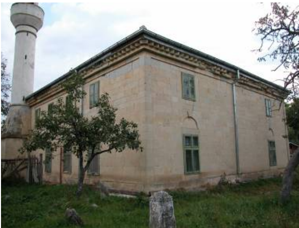
Oblique view, right and qibla walls. Note placement of stones to create pediments and architraves in relief. Also note recently emplaced gutters and drain pipes.
