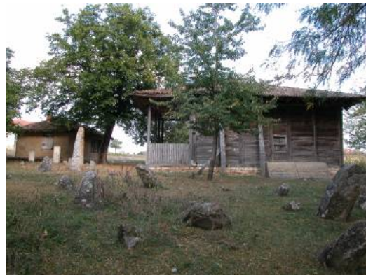
Lateral view, right side. In the foreground, the remains of the cemetery. At the far left, the former mehtep . Note the older wooden buttressing of the wall of mosque and more recent brick and concrete reinforcement at the base of the wall.
