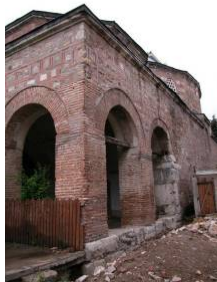
Close-up of piers. Note that the piers are of brick. Also note the high-quality of the cloisonné work and that the portico and sanctuary are of a single piece. Signs of excavation work are visible in the foreground.
