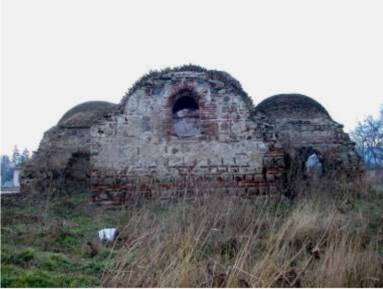
Rear view. At the center: the rear or mihrab wall of the mosque sanctuary. Note that its window opening is original. At the right: The left-hand chamber. Note large holes knocked through the walls of the chamber.
