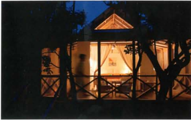
Typical cottage in the resort we can see is very open to allow light and ventilation. This is emphasized in the roof condition and in plan
