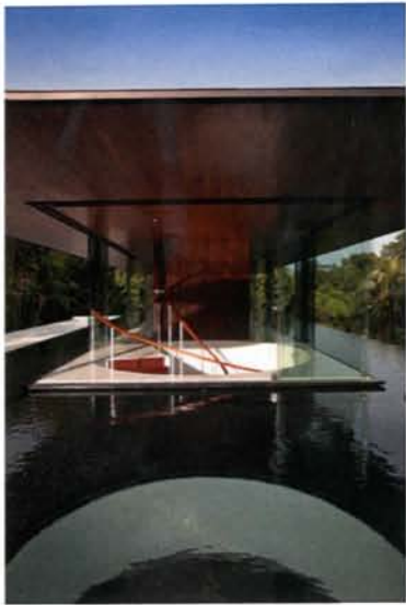
water level veiw of skylight
