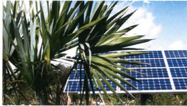
Landscaping used to minimize the visual impact of the pv panels, also one can see the structure used to hold the panels in made to minimize the impact on the ground
