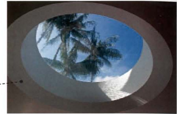
veiw of skylight fom above water level
