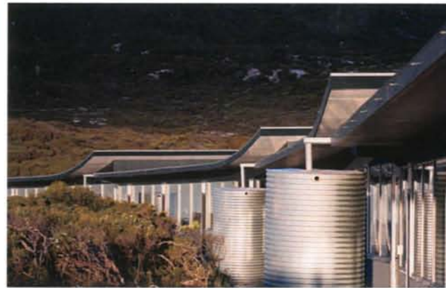
Detail of water collection roof Configuration with low pitched roofs and aluminum tanks on the end
