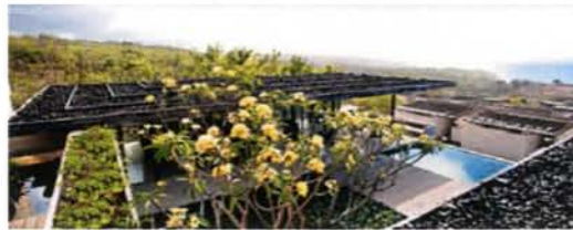
view of roofs
