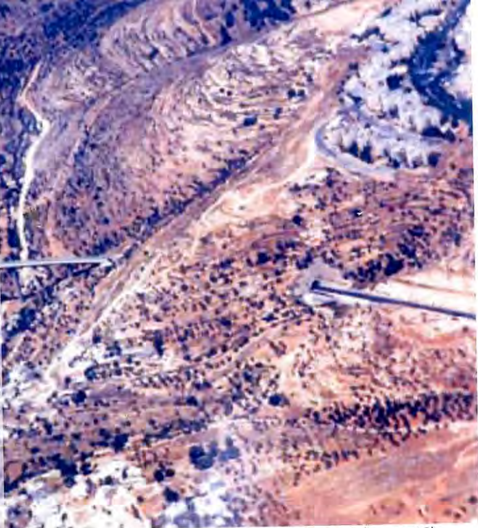
tunnels road (image 18)
