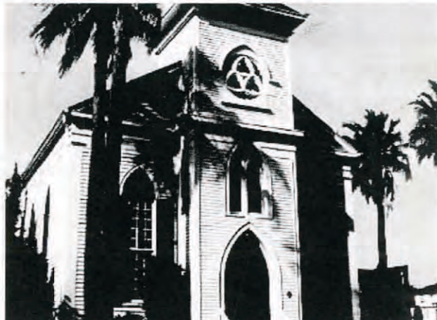
St. Joseph's Church The oldest German Catholic Church in Texas and the oldest wooden church building in Galveston, St. Joseph's was built by German Immigrants in 1859-60. The building is a simple wooden gothic revival structure, rectangular with a square bell tower with trefoil window. The softly painted interior features a coffered ceiling with painted quatrefoils and other gothic symbols, plaster of Paris.
