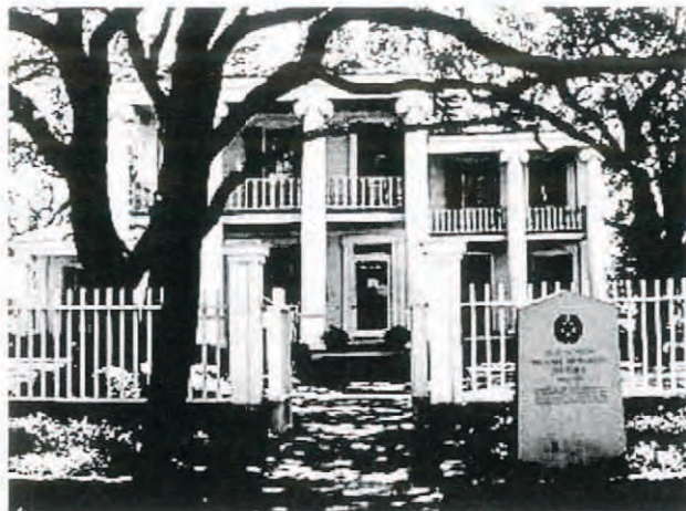
Michel B. Menard House The house, built in 1838 and the oldest on the island, is in the Greek revival style.
