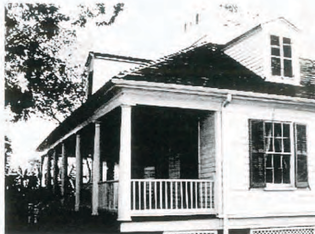
Samuel May Williams This rare combination of Creole-plantation and New England architectural styles was built in 1838 for Samuel May Williams, secretary to Stephen F. Austin and founder of the Texas Navy.
