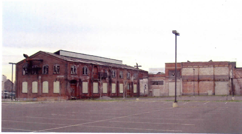
-Building #1 Sits on the north end of the site and at the site's only major intersection. It has the largest footprint of the three buildings. Portion of built in 1808 but majority was built in 1930.
