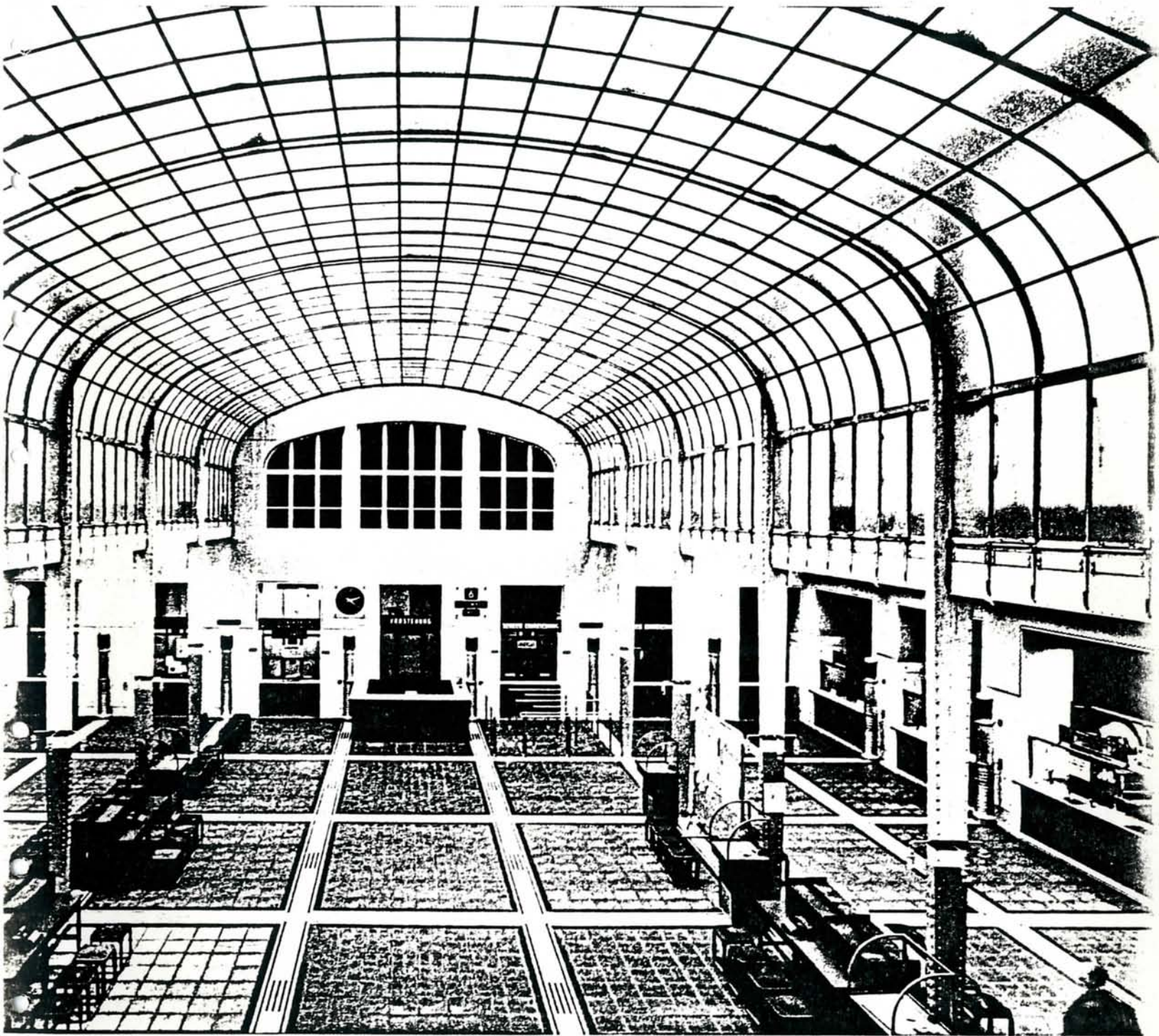
Ill. 189. Post Office Savings Bank: Counter section as seen from the vestibule of the governor's office. The glass span roof shown in Ill. 184 is situated immediately above the glass ceiling. The rooms beneath the counter section were lit through the glazed panels in the floor.
