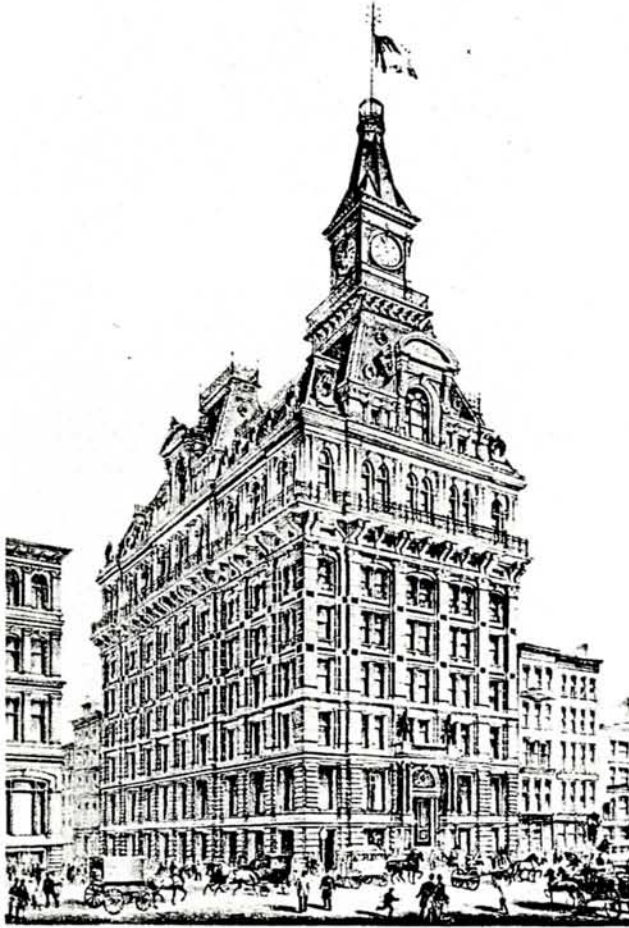
13.25 New York, Western Union Building, 1873-75, by G. B. Post
