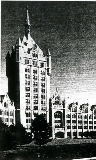
delaware and hudson building and alban evening journal building
