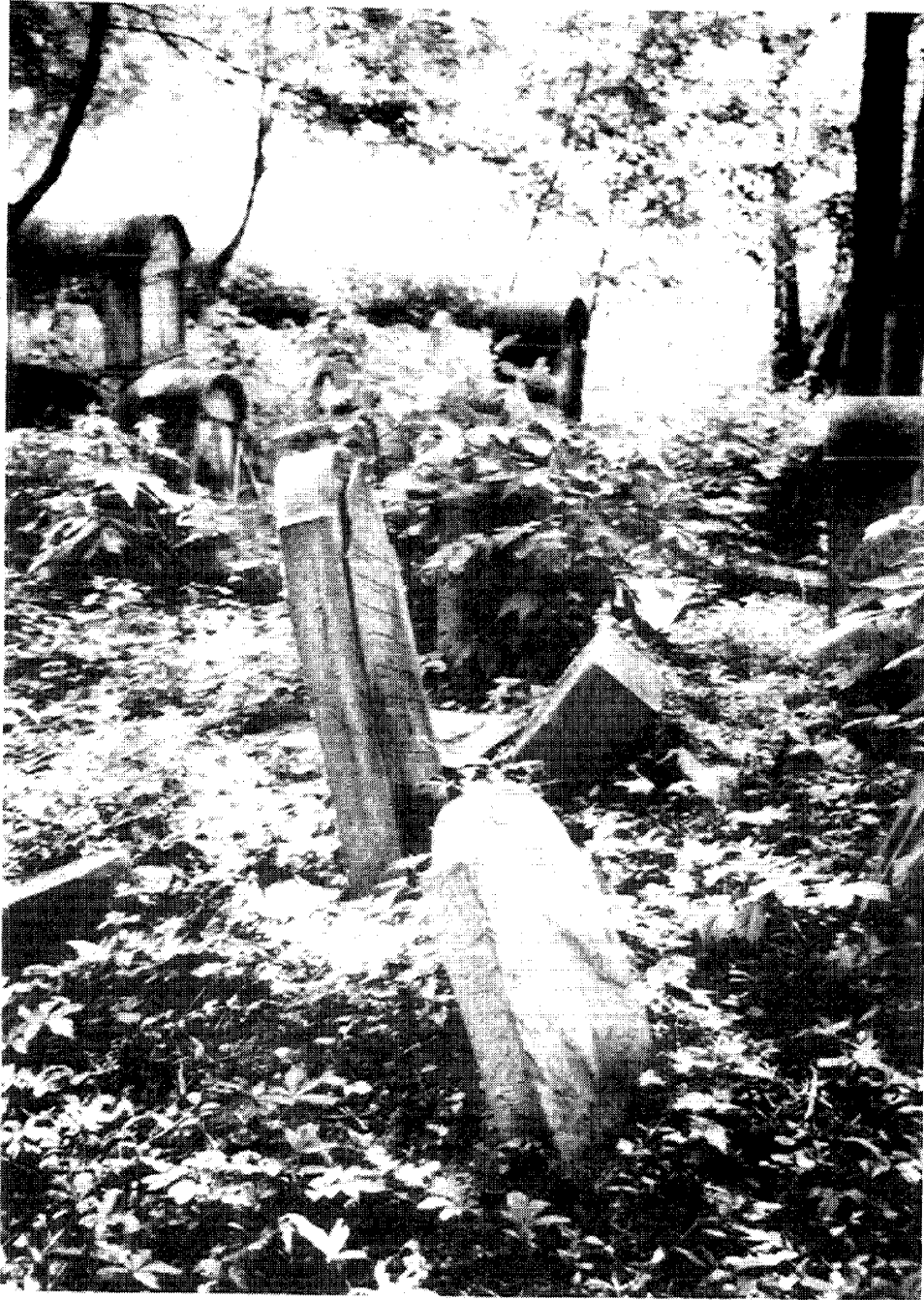
Tarnow. Many stones, especially those cut from limestone, sandstone, slate and marble suffer from pollution or the weather. Carved surfaces erode and crumble, whole sheets of stone peel away. (photo: S. Gruber 6/93)
