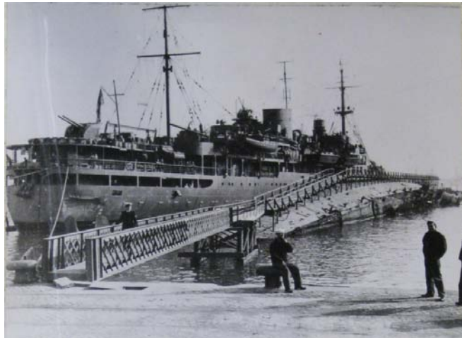
Figure 23: Pier Extended Over Sunken Ship at Naples 601
