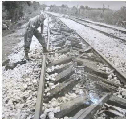
Figure 28: Damaged Ties 653
