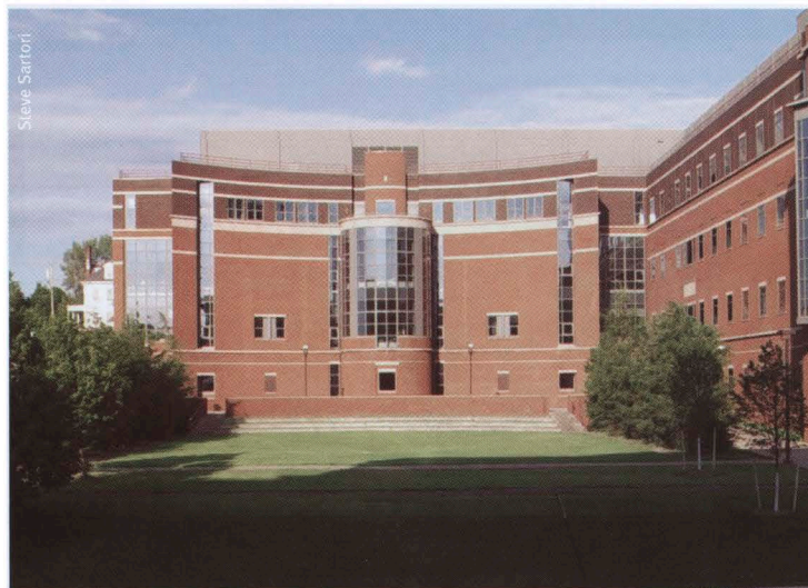
An addition to the Center for Science and Technology will become a new Life Sciences Center.
