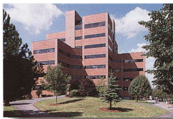
CROUSE-HINDS SCHOOL OF MANAGEMENT BUILDING
