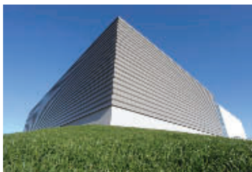
Constructed in six months, the 12,000 square-foot Green Data Center is located on SU's South Campus.
