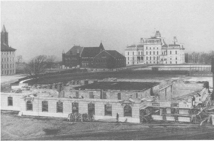
Fig. 5. Carnegie Building under construction.
