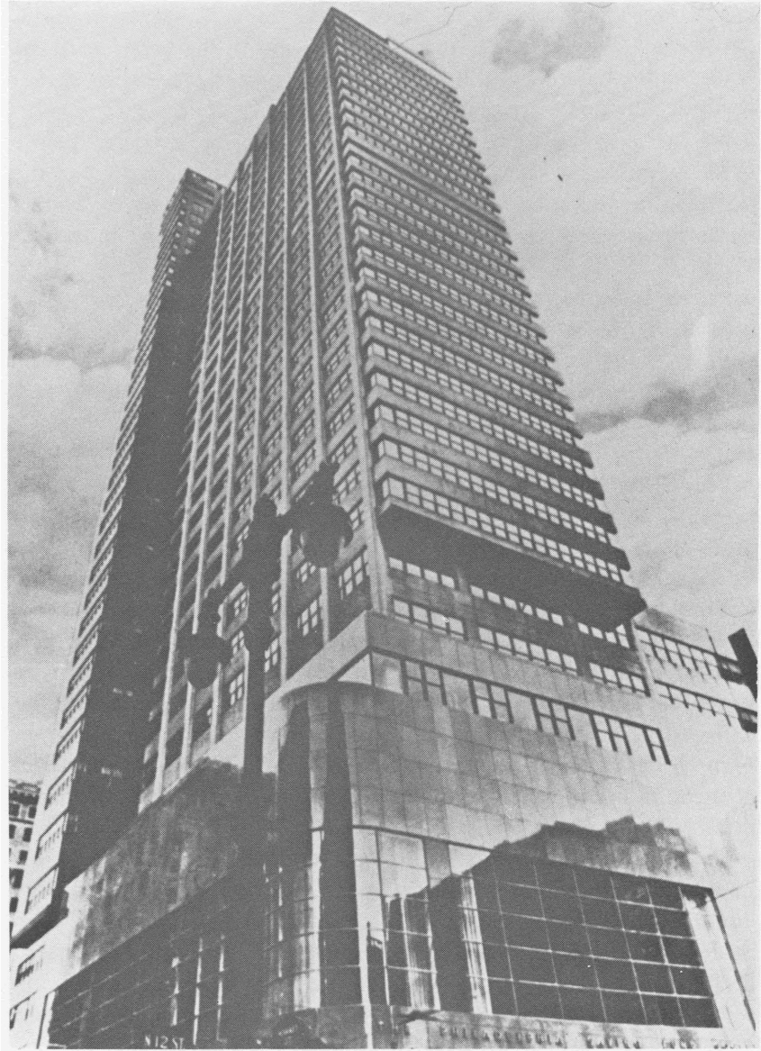
Fig. 2. Howe and Lescaze, Philadelphia Saving Fund Society, 1929-32, north and east elevation (R. T. Donner).
