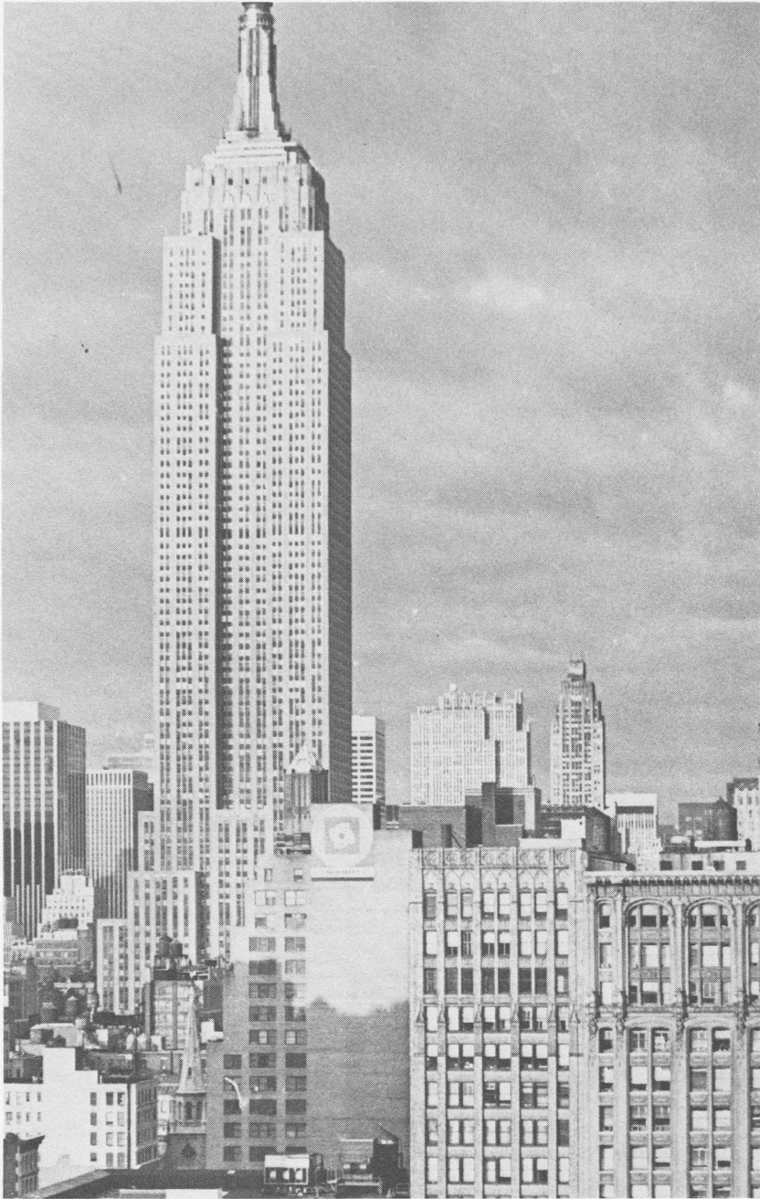
Fig. 7. Shreve, Lamb and Harmon, Empire State Building, 1930-31 (author).
