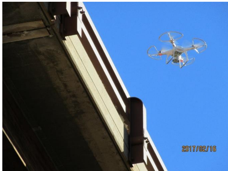
Fig. 4-3. Selected DJI Phantom 4 UAV flying near the Keystone Wye Bridge (image captured by Junwon Seo).
