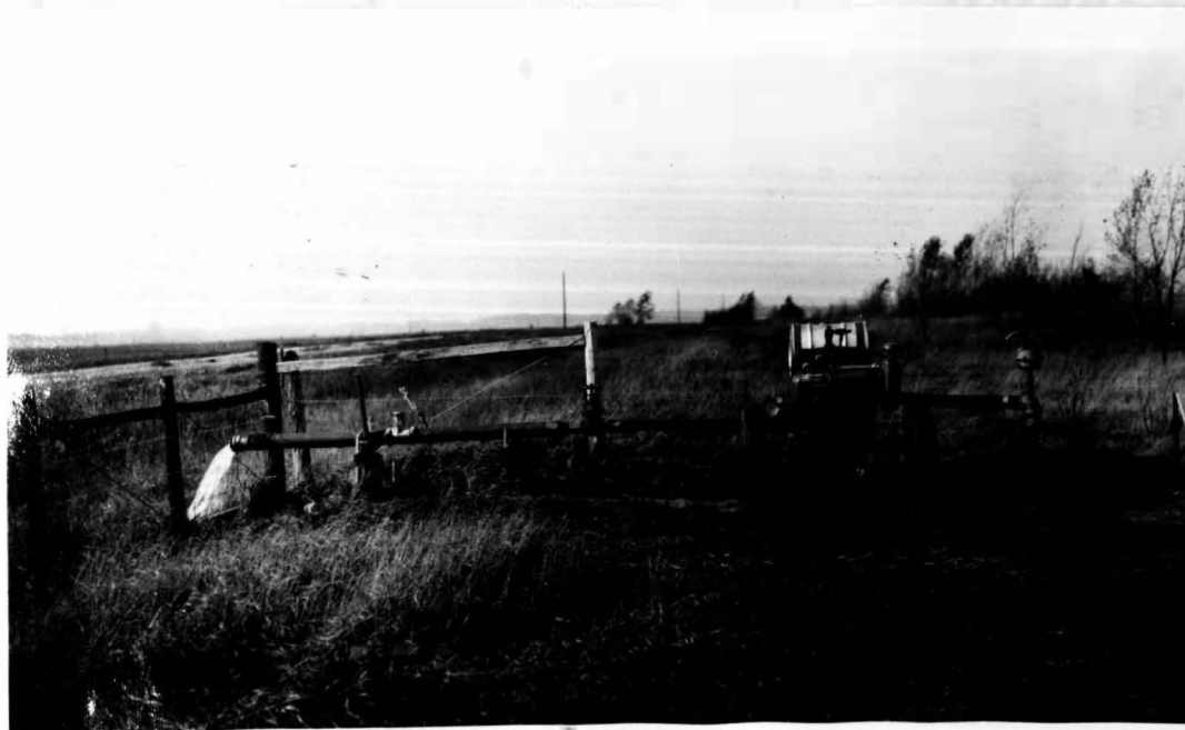
Figure 7. A Discharge of over 80 Gallons Per Minute
