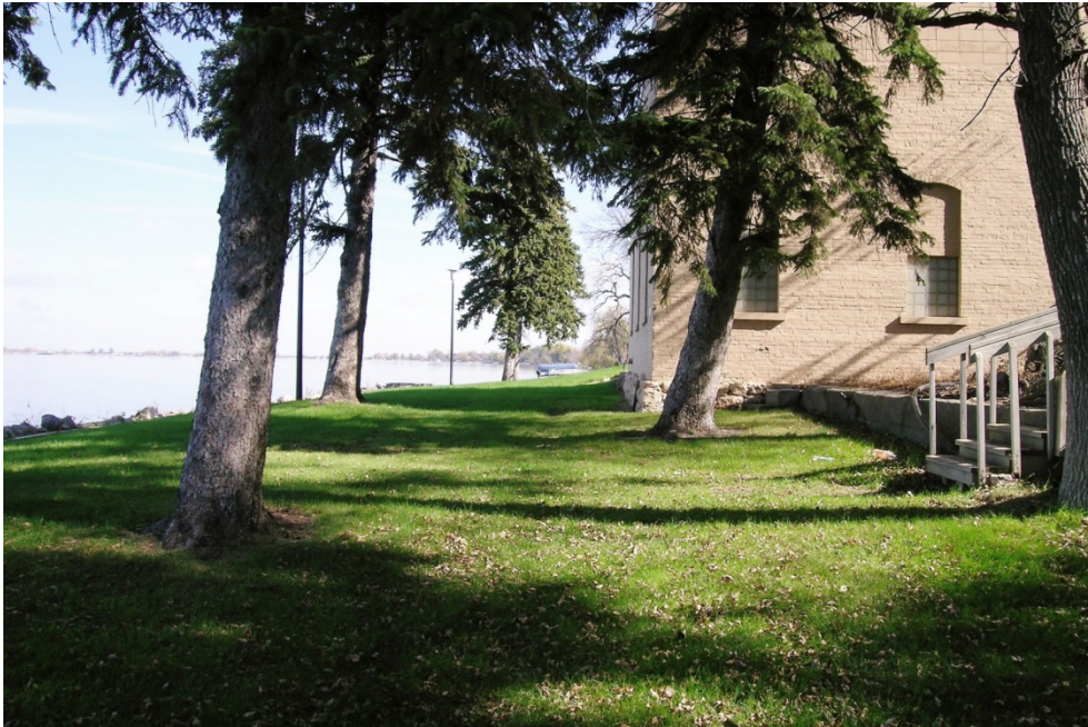
12. and 13. Pumping station, same views, 12 October 2007. Note the altered shoreline in comparison to photos 9, 10, and 11 (Appendix A, Figure 1, "c").
