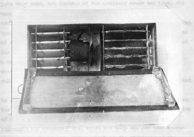
PLATE III - Top view of humidifier with cover removed.
