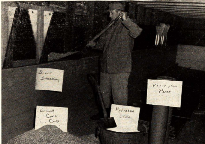
Fig. 1. Insulating material is filled between studs.
