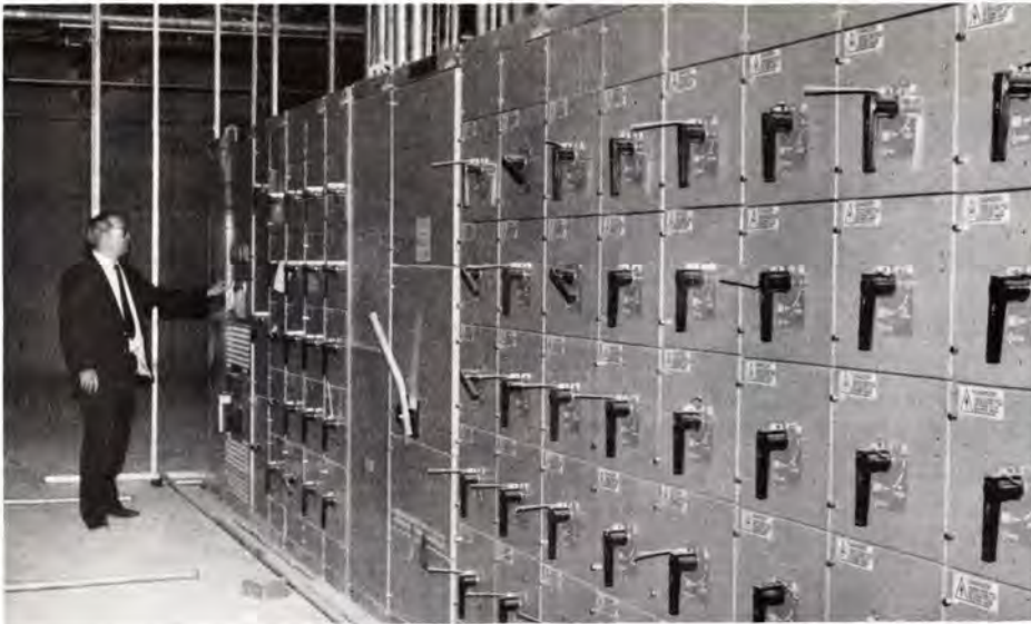
Facing page: The atrium entrance of the Northern Plains Biostress Lab has not been enclosed at date of this photo. The atrium looks west. Above: Ken Schmidt, utilities engineer and project coordinator, examines the main electrical distribution panel in the basement of the lab.
