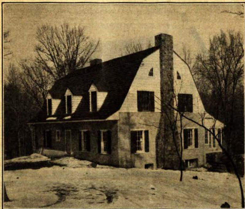
FIG. 2.—A house near Washington, D. C. The first-story walls are of rammed earth resting on a foundation of concrete blocks
