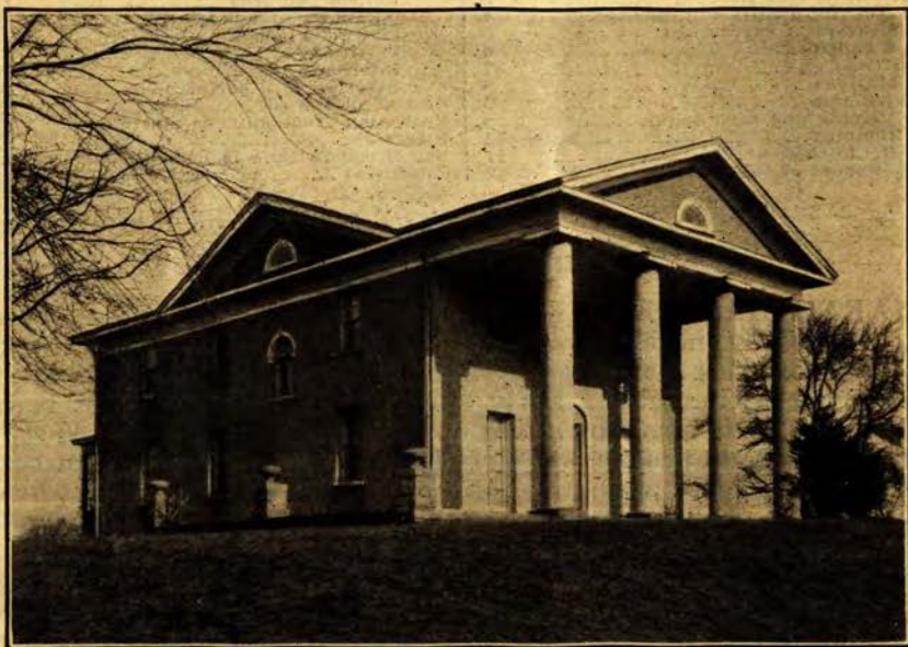
FIG. 1.—A house now standing in Washington, D. C., the main portion of which was built of rammed earth in 1773. The portico and rooms at rear have been added in recent years
