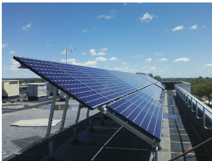
Figure 2.13. Solar panels (Evergreen ES-A-205-FA3) on the rooftop of Daktronics Engineering Hall, SDSU.
