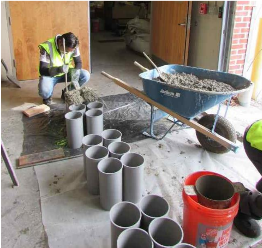
Figure 2-5. Casting of concrete cylinders
