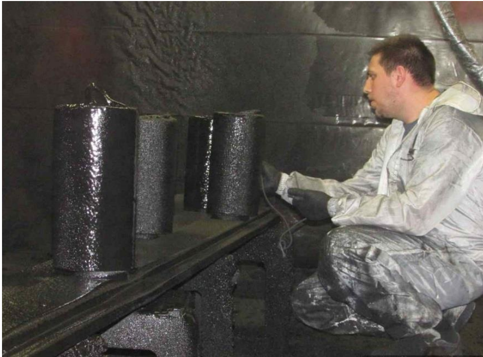
Figure 2-9. Rubber thickness measurement
