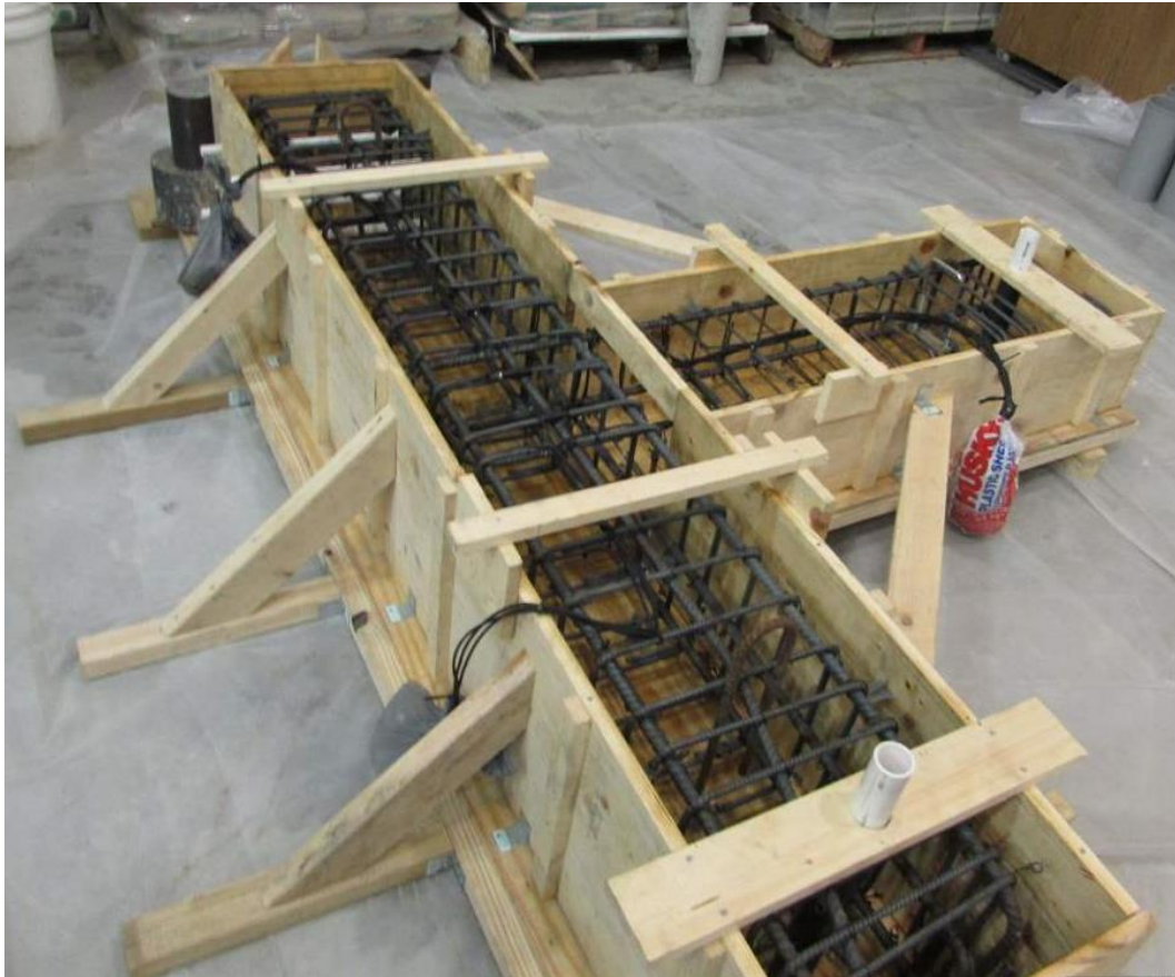
Figure 4-16. Steel cage and formwork
