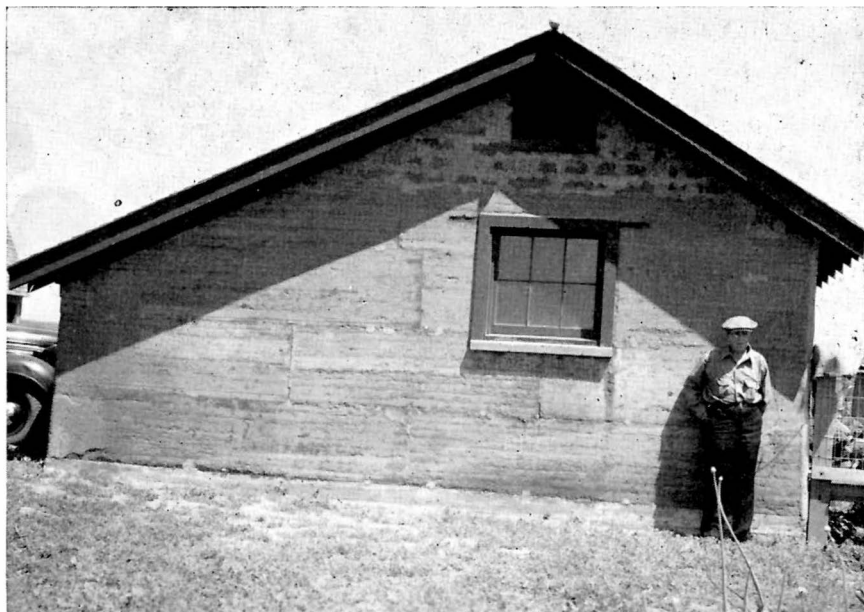
The rammed earth poultry house before a stucco coat was applied. Standing in front of the building is Jacob Weller, who supervised the building of the house in 1938
