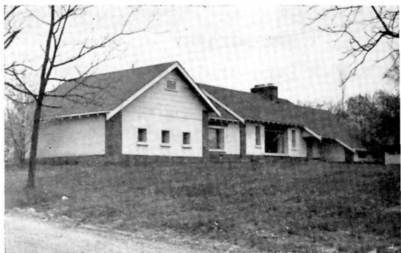
This rammed earth home is located at Salem, Missouri.
