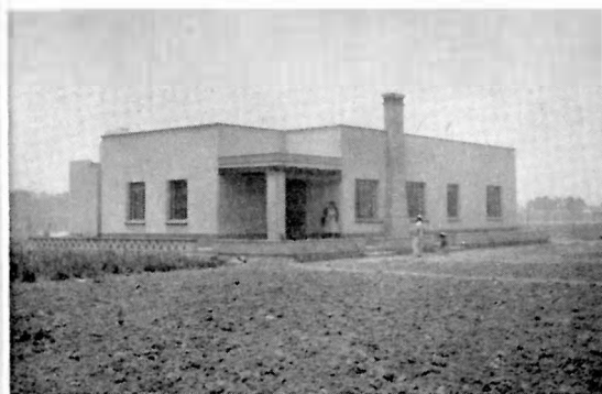
A rammed earth home in Mexico is shown in this picture.
