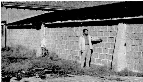
Monolithic rammed earth barn with stucco cover and shed of uncovered block, built in 1936-37 at the Pine Ridge, South Dakota, Indian School, looks like this in 1959.
