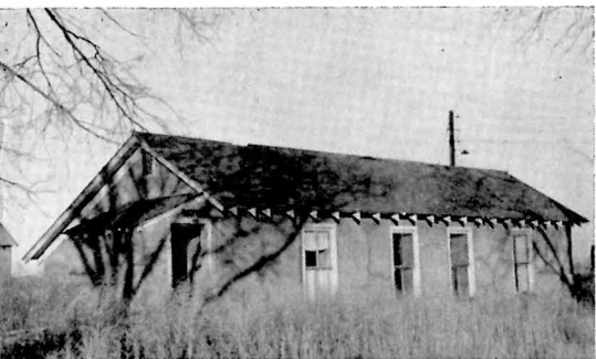
This photograph was taken in 1959 of a poultry house at Flandreau, South Dakota. It was built in 1939 and used as a residence until 1957.
