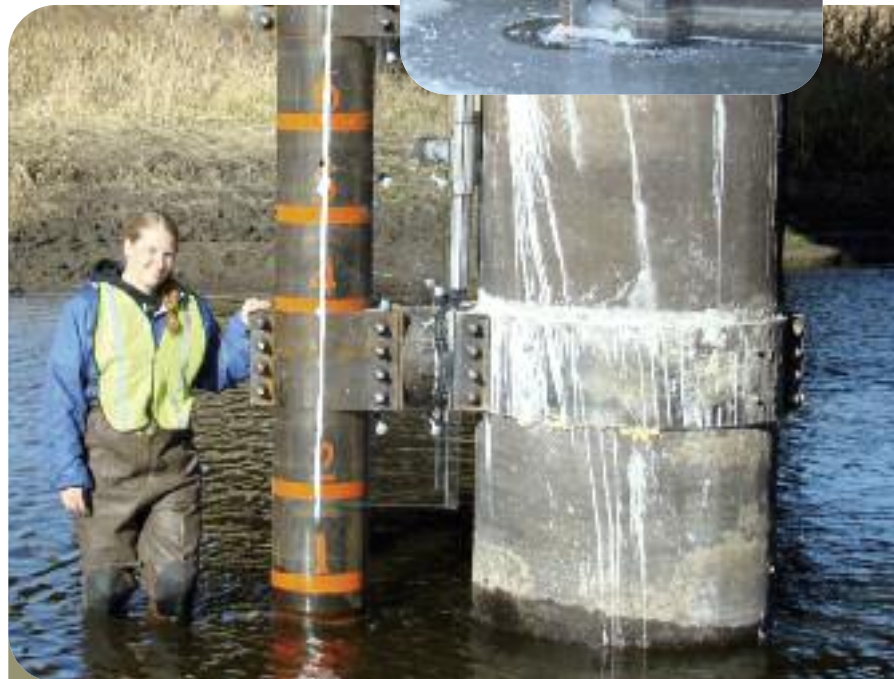
Top: Ice hugs a bridge pier and an attached measuring device in the James River east of Huron. The device is used in a project to calculate ice load.
