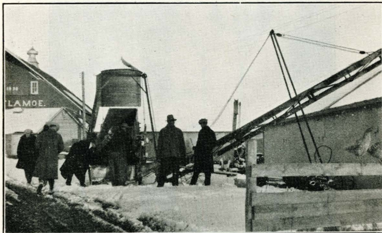
FIG. 7.—ELEVATING CORN INTO THE CRIB BY ELECTRICITY
