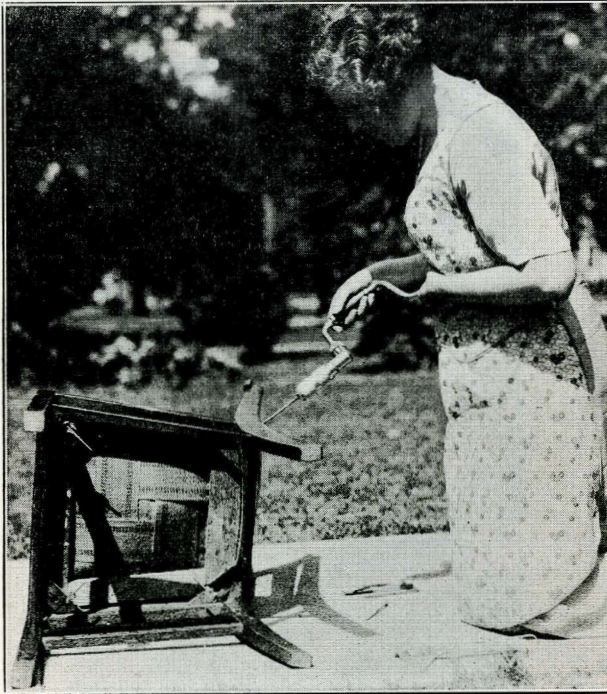
Fig. 1.—Holes are bored diagonally through the legs.
