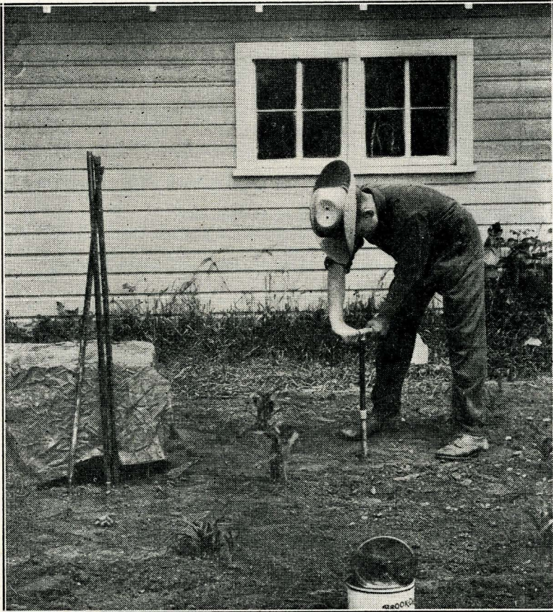
Fig. 1.—TESTING THE LOCATION FOR A PIT SILO
