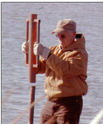
Metal pipes were driven into the marsh substrate from a boat or through a hole cut in the ice and used as support for cylinder and basket nesting structures (Paul Mammenga in photo).
