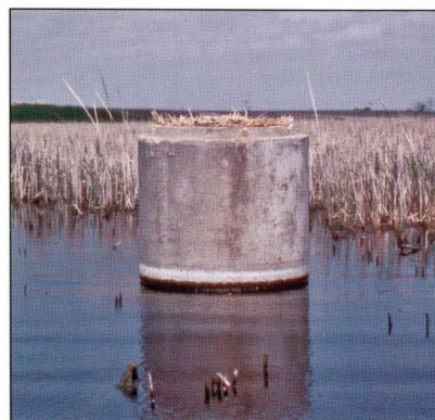
The first experimentation with earth-filled concrete culverts was conducted in the 1970s in North Dakota and showed promising results for nesting mallards in years when Canada geese were not using the structures (Higgins et al. 1986).
