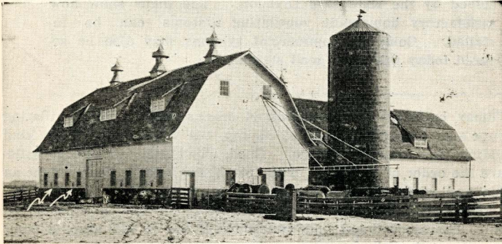
Fig. 3—A barn in Minnehaha County, South Dakota. Note the many fresh air inlets. Without them your ventilating system is worthless.
