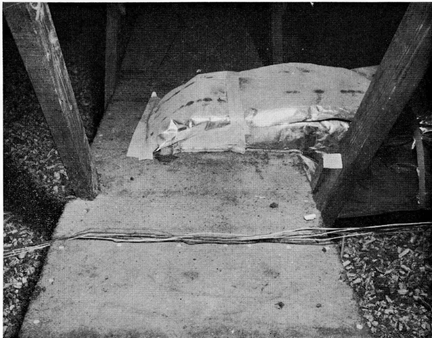
Figure 9. Typical duct construction.
