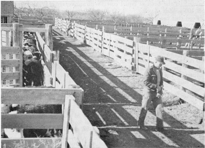
Corrals and working chute at the Range Field Station, Cottonwood. The building to the left is the scale house. This arrangement permits use of the chute without the cattle having to cross the scale unless so desired.
