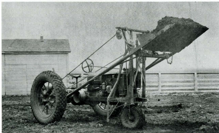
Fig. 3. The loader in position to dump into the spreader.
