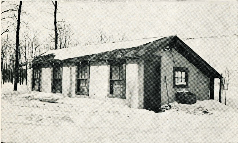
Fig. 3. Ordinary Stuccos Have Been Successful on Rammed Earth Walls.
