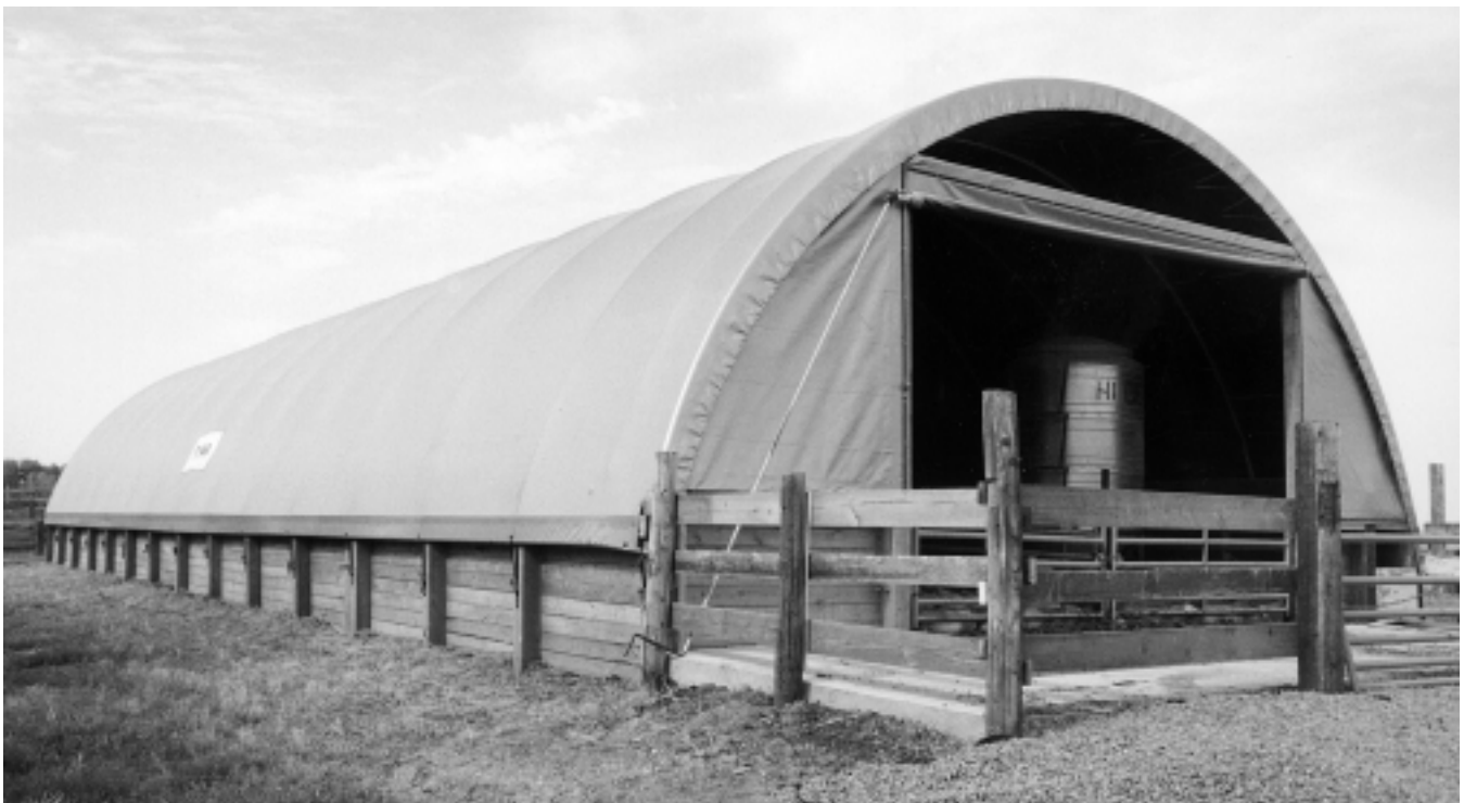
The hoop barn at the Southeast Experiment Farm at Beresford is an economical shelter for finishing hogs or other uses. Just roll in the big bales of straw, says Bob Berg, farm manager, and the pigs take care of spreading and rearranging the bedding to their liking. This hoop barn went up in 1998 for $15,000.
