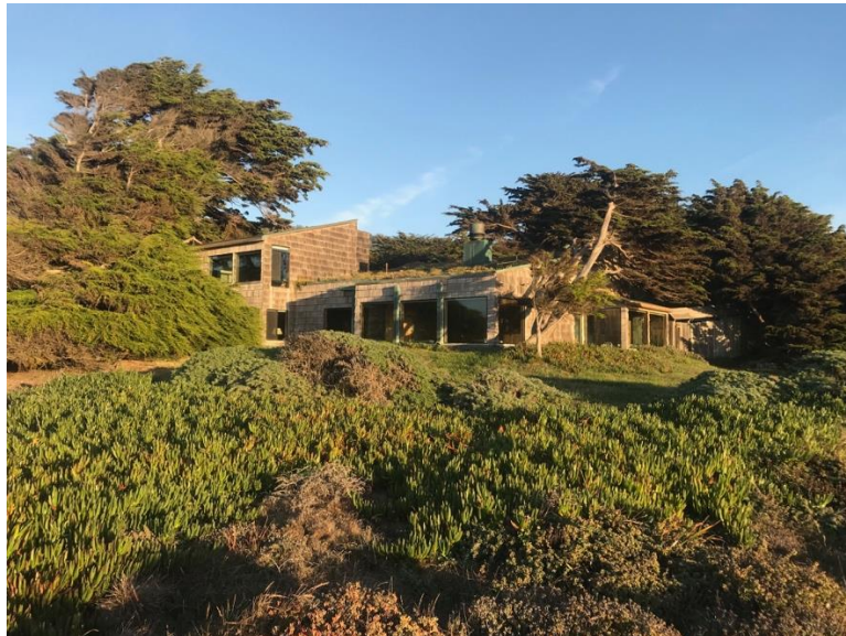
Figure 8 Hedgerow House with Sod Roof, 2018
