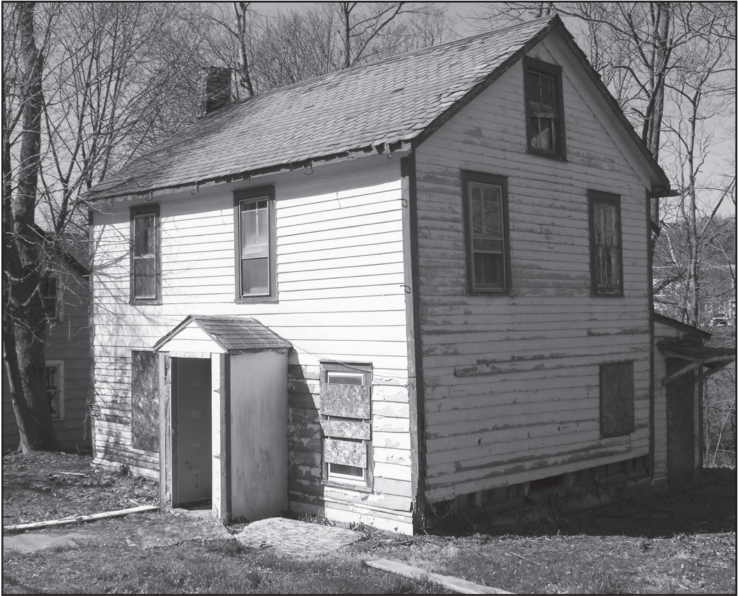
Figure 2. Cooper-Mann House prior to demolition. (Photo by Michael Tomkins, 2009.)
