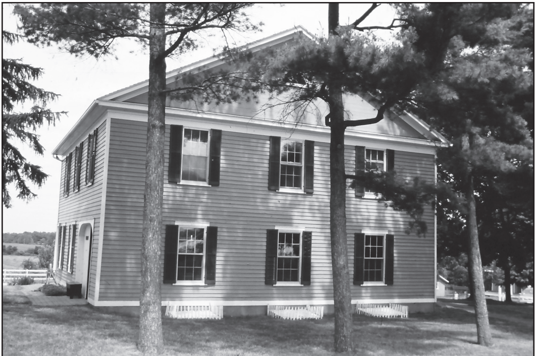
Figure 2. The original house at Rose Hill, constructed for Robert Rose in 1809. This building was moved off its original foundation during the renovation of the estate in the late 1830s, when it was converted into a carriage house. It is missing an attached kitchen that remains part of the second house. (Photo by James A. Delle, 1998.)
