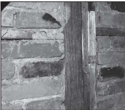
Figure 18. Interior wall of the Jean Nicholas House, featuring hewn timbers and roughly made brick masonry. (Photo by James A. Delle, 2007.)
