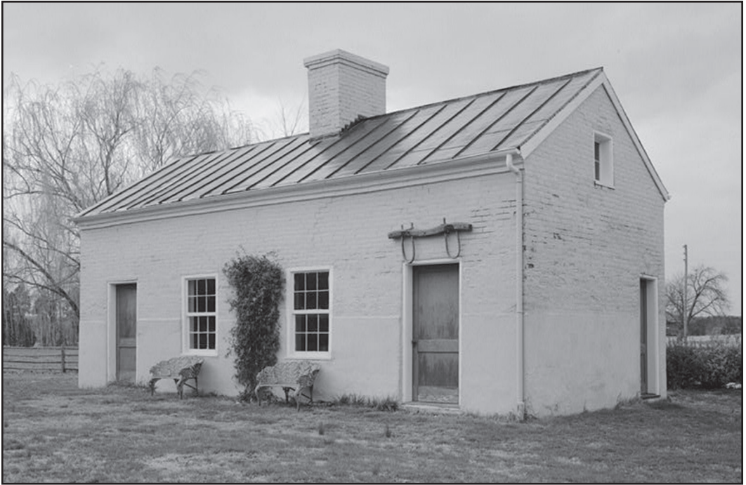
Figure 14. Nineteenth-century slave quarter, Westend Plantation, Louisa County, Virginia, another story-and-a-half brick duplex. (Library of Congress, Prints and Photographs Division, digital archive of HABS, HABS VA,55-TREV.V,14C—2, accessed April 15, 2013.)
