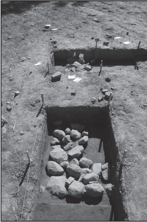
Figure 9: Segments of the dry-laid foundation of the kitchen extension, including the northwest corner ( bottom of image). (Photo by James A. Delle, 2007.)
