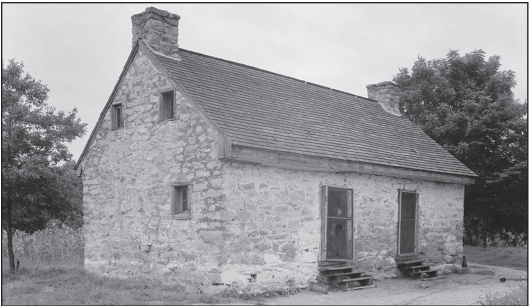
Figure 13. Nineteenth-century slave quarter at Berry Hill Plantation, Halifax County, Virginia. Note that this structure is also a story-and-a-half duplex, though rendered in stone. (Library of Congress, Prints and Photographs Division, digital archive of HABS, HABS VA,42-BOSTS.V,1-17, accessed April 15, 2013.)
