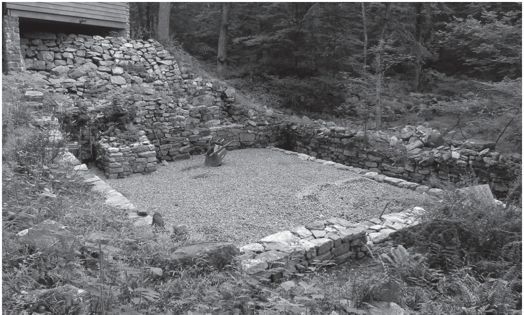
Figure 15. The stabilized forge site as it currently appears.
