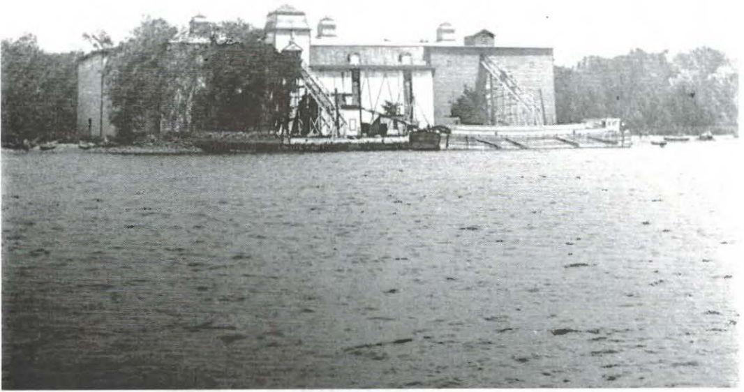
Figure 11. Ice House Site C (the Van Orden, Vanderpool, & Sherman Ice House) depicted in a photograph apparently taken at the turn of the century. The portion of the structure at the right is a post-1896 extension. (Courtesy of the Vedder Memorial Library, Greene County Historical Society.)
