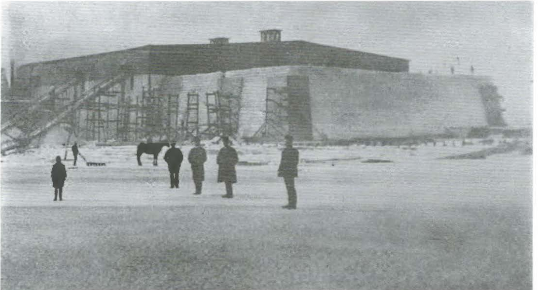
Figure 5. Undated photograph of Hudson River ice house with additional ice stacked beside it. Visible at the left side of the photograph are the steam-powered elevators for hoisting ice cakes from the river and the wooden "runs" that carried the ice cakes through the vertical doors into various internal rooms. (Courtesy of the Vedder Memorial Library, Greene County Historical Society.)
