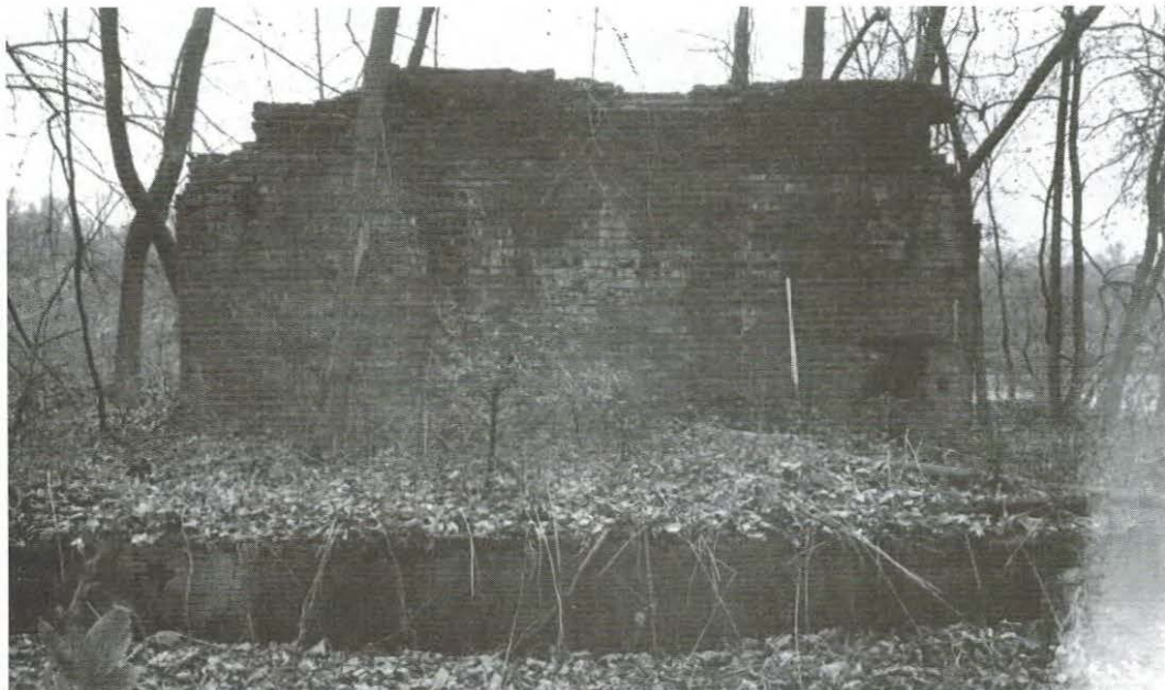
Figure 17. Remains of Ice House Site B (the P. McCabe & Co. Ice House) powerhouse. In the background is the narrow brick structure, designated Feature A, which may have housed the steam engine boiler and firebox. Coal was probably shoveled in through the opening visible at the right end of the structure's exterior wall. The view is towards the east.
