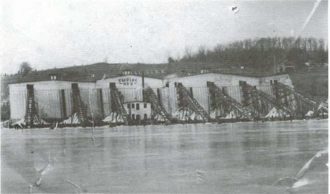
Figure 21. Substantial variation existed among Hudson River ice houses in the configuration of elevators used to load ice. Here, in an undated photograph of the Empire Number 2 Ice House at Catskill, NY, a separate elevator is located in front of each door. (Courtesy of the Vedder Memorial Library, Greene County Historical Society.)
