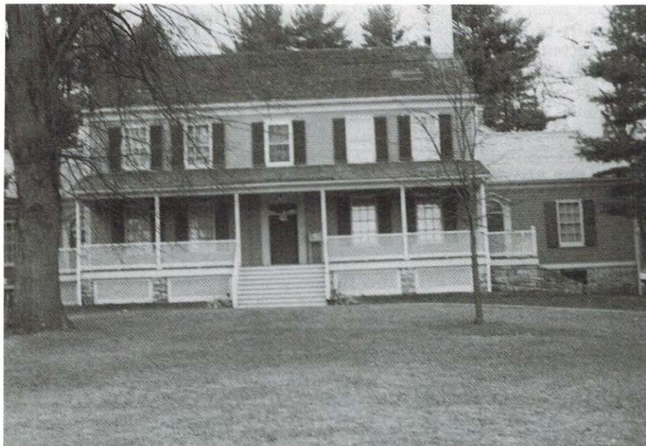
Figure 2. John Jay Homestead as seen from the south.
