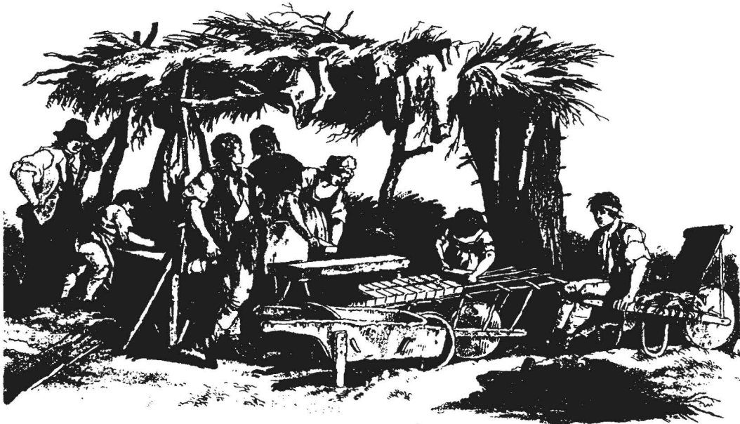
Figure 3. Top: early 19th-century drawing of brickmaking operations. Note the horse-powered pug mill on the upper right (Pyne 1977: plate 106). Bottom: early 19th-century drawing of the molding and drying of brick. Note the heaps of clay, freshly molded bricks, and the temporary nature of the entire operation (Pyne 1977: plate 105).
