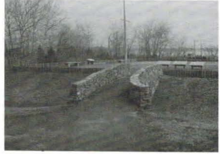
Figure 20. A view (facing east) of the granite walls and walkway leading to the fort exhibit in the Fort Saybrook Monument Park. (Photograph by H. Juli, 1990.)
