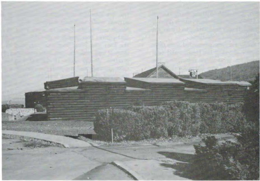
Figure 6. The southwest bastion of the reconstructed fort in the fall of 1993, lying atop the remains of the original 1755–1757 fort. Lake George is in the background on the left.
