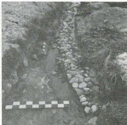
Figure 10. The French drain protecting the Woodworth farmhouse and barn. This view (facing south) shows the drain as exposed in Trench 9, on the eastern side of the site.
